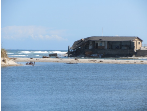
Pea Island NWR building damaged by Hurricane Irene
